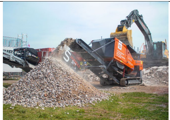
Construction waste processing with the IMPAKTOR 250 evo live at RecyclingAKTIV 2022
